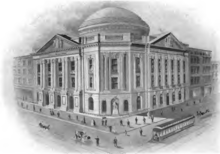
CLEVELAND TRUST CO., CLEVELAND, OHIO. The New Bank Building Now Under Construction.
